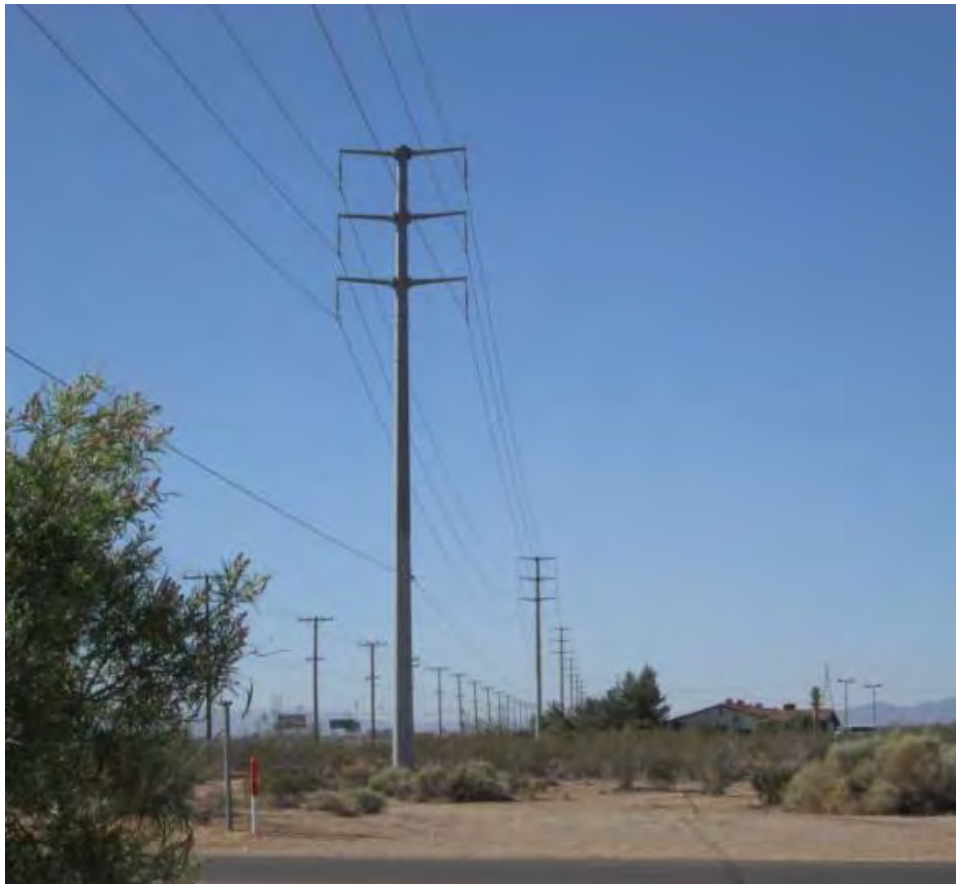
View looking south from intersection of Air Expressway Boulevard and US 395.
