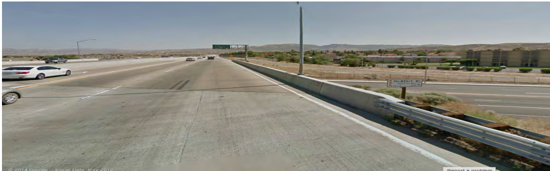
Figure 3.1.7-7 KV #2 Existing View
