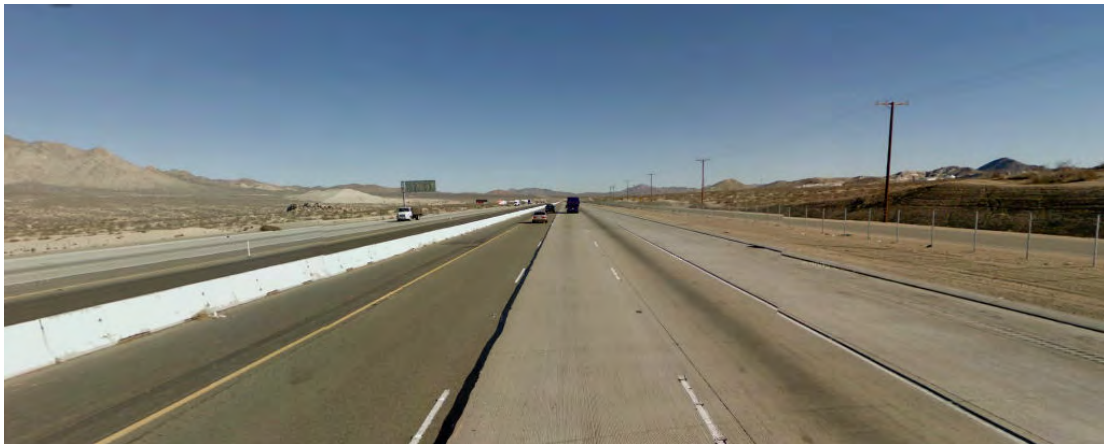
Figure 3.1.7-48 KV #21 Existing View
