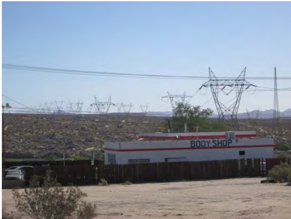
View looking east across building on National Old Trails Highway/Route 66.
