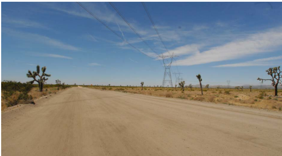
Figure 3.1.7-34 KV #14 Existing View
