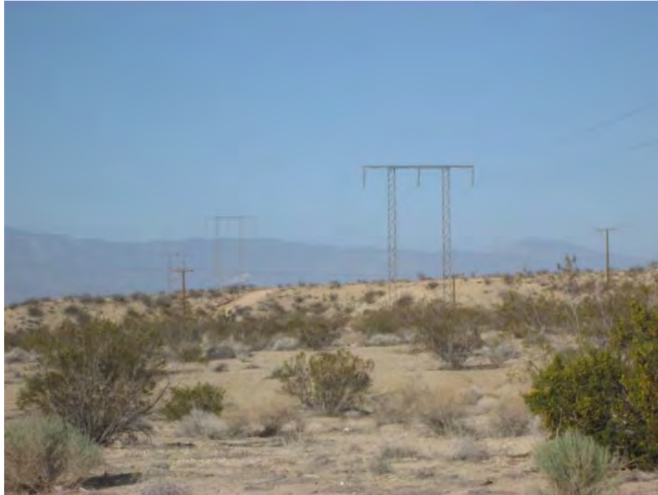
View looking west from County Refuse Disposal Site Road (off of Stoddard Wells Road).
